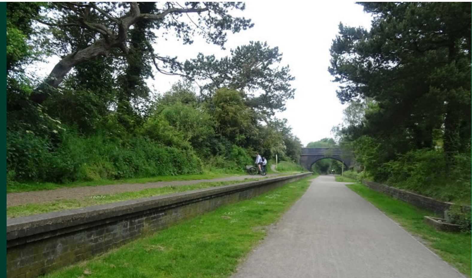
Segregated rural cycleway
